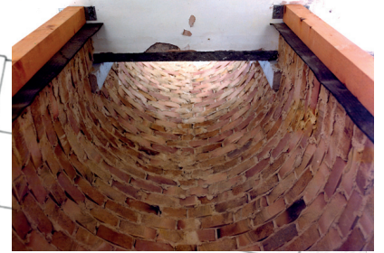
The over-cladding in wood and brick could be made by any builder. It was cheap, durable and maintenance-free.
